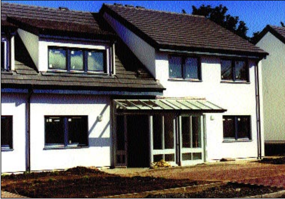
Figure 6.3 Solar porches as entrances help reduce air leakage
