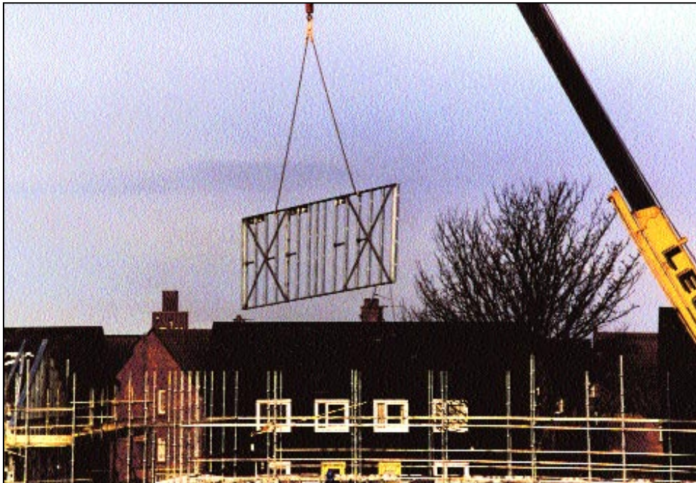
Figure 6.2 Steel construction increases efficiency in housing construction.
