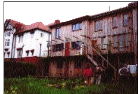
Figure 6.4 This housing has used untreated larch timber for cladding (Gledhill Leeds).
